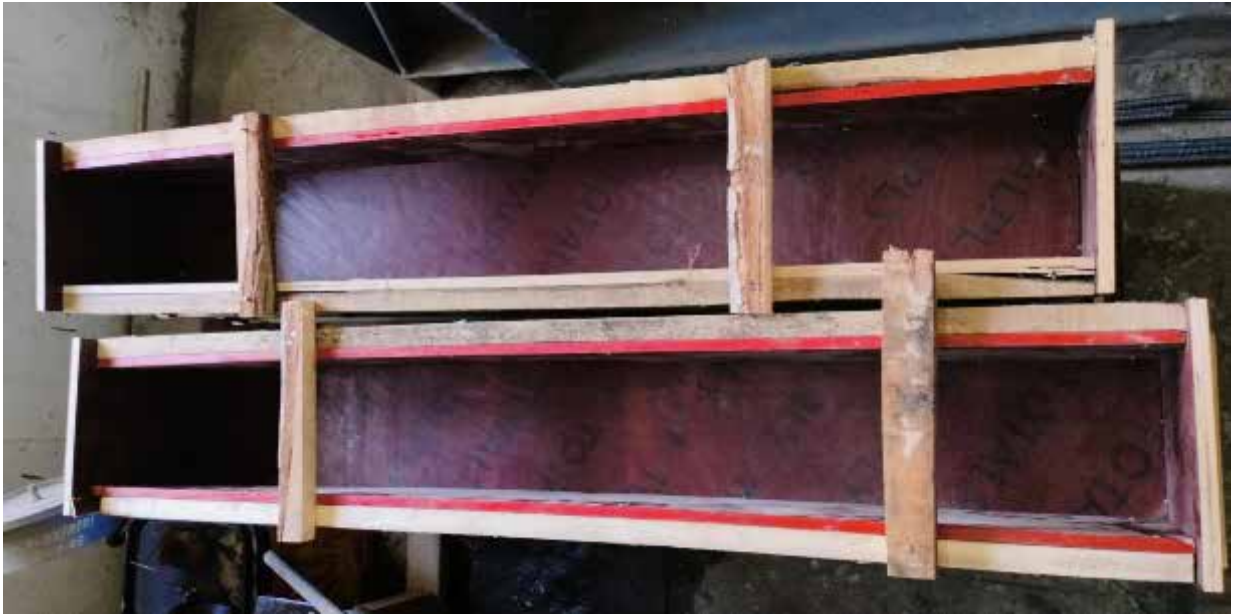
Figure.1 Mould preparation for casting of beam.
