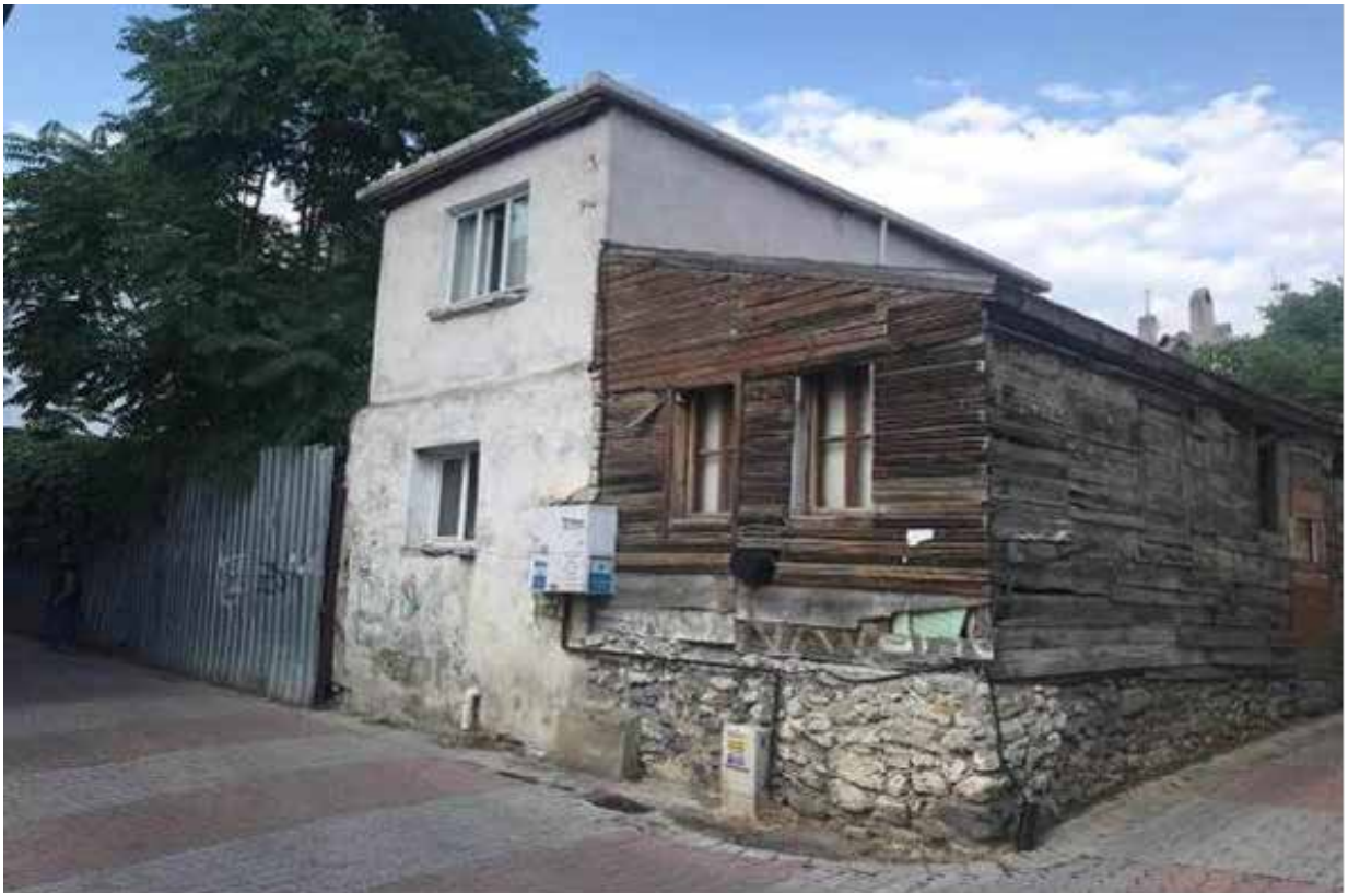
Fig 3 View from "Cami arası Row", Source: Arch. SEDES, F.
