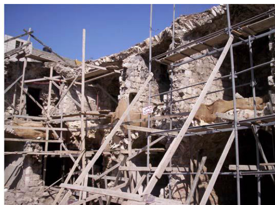
Figure 16. To the right business consolidation by wooden struts of the northern facade of Khan, to the left to strengthen the roof of one of the rooms in the building from the inside by pillars (3).
