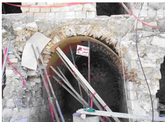
Figure 16. To the right business consolidation by wooden struts of the northern facade of Khan, to the left to strengthen the roof of one of the rooms in the building from the inside by pillars (3).
